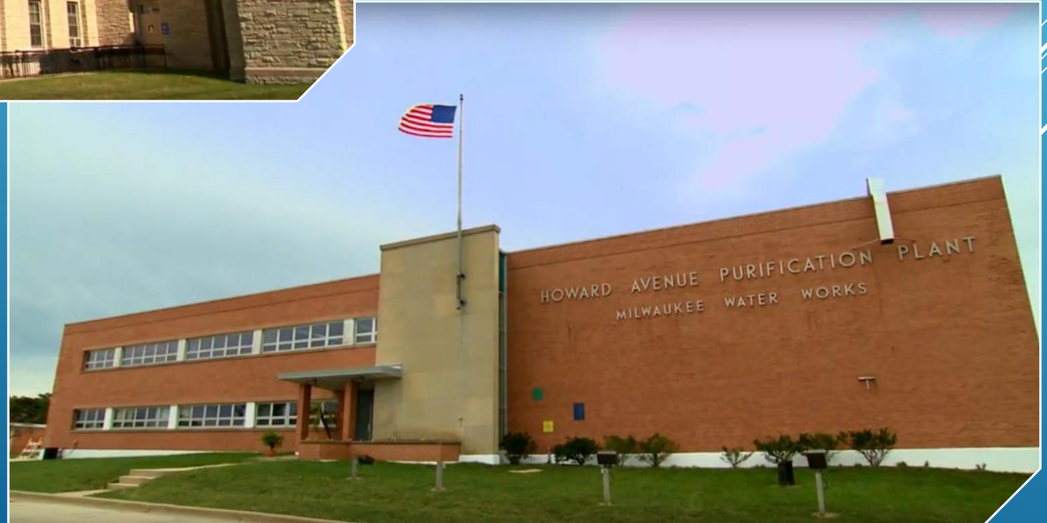
Howard Ave. Purification Plant
