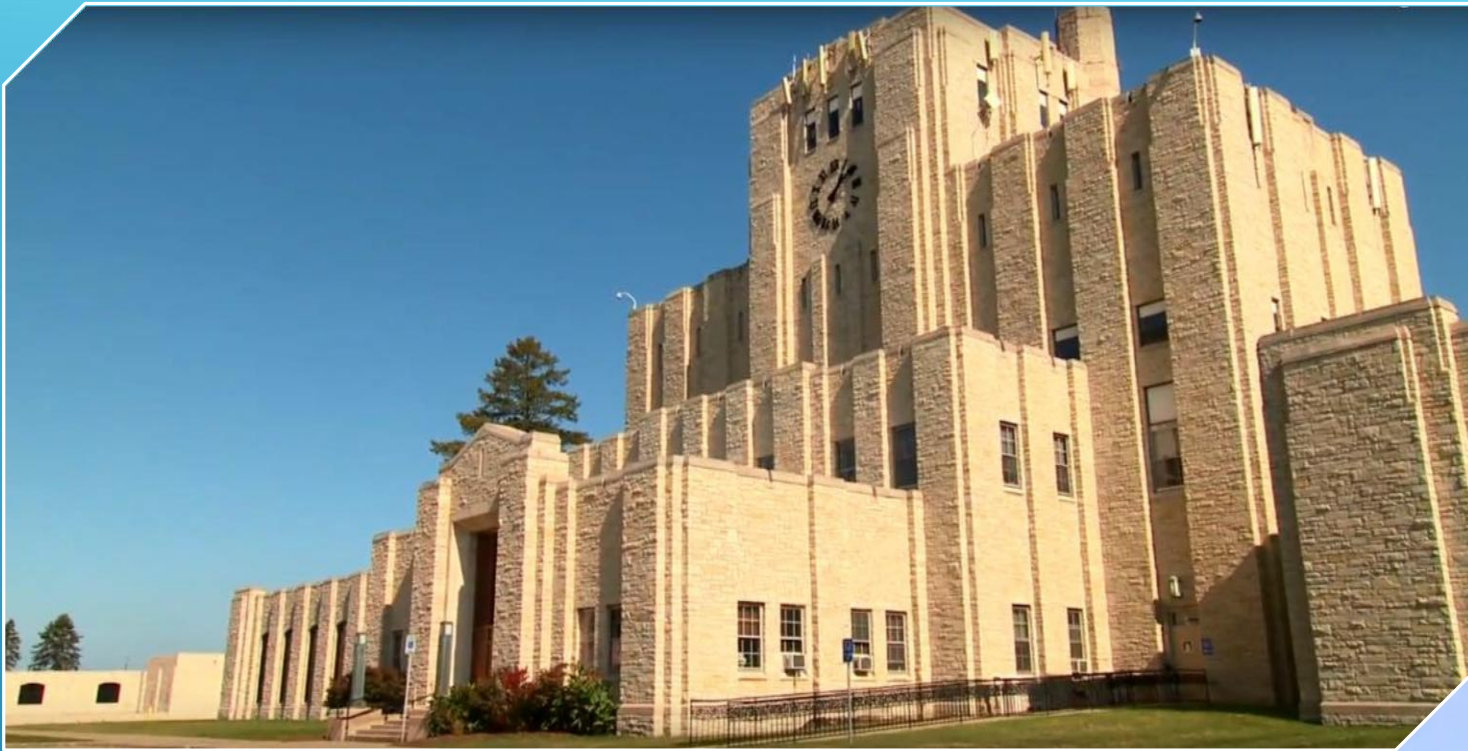
Linnwood Purification Plant
