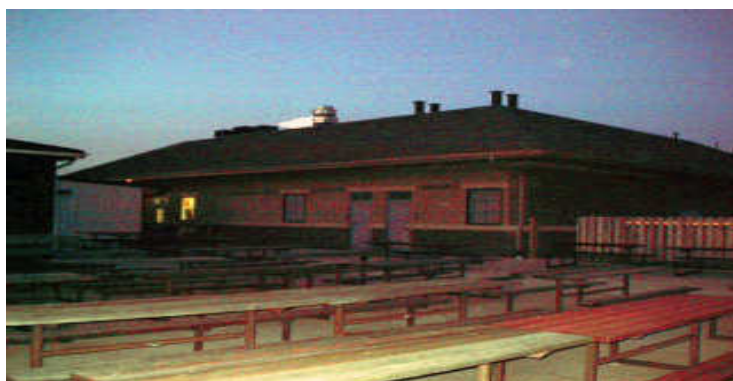
This is a view of the Kitchen & Bathroom building
